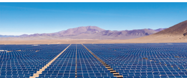
Hitachi Energy: the Al Kharsaah solar power plant in Qatar.
